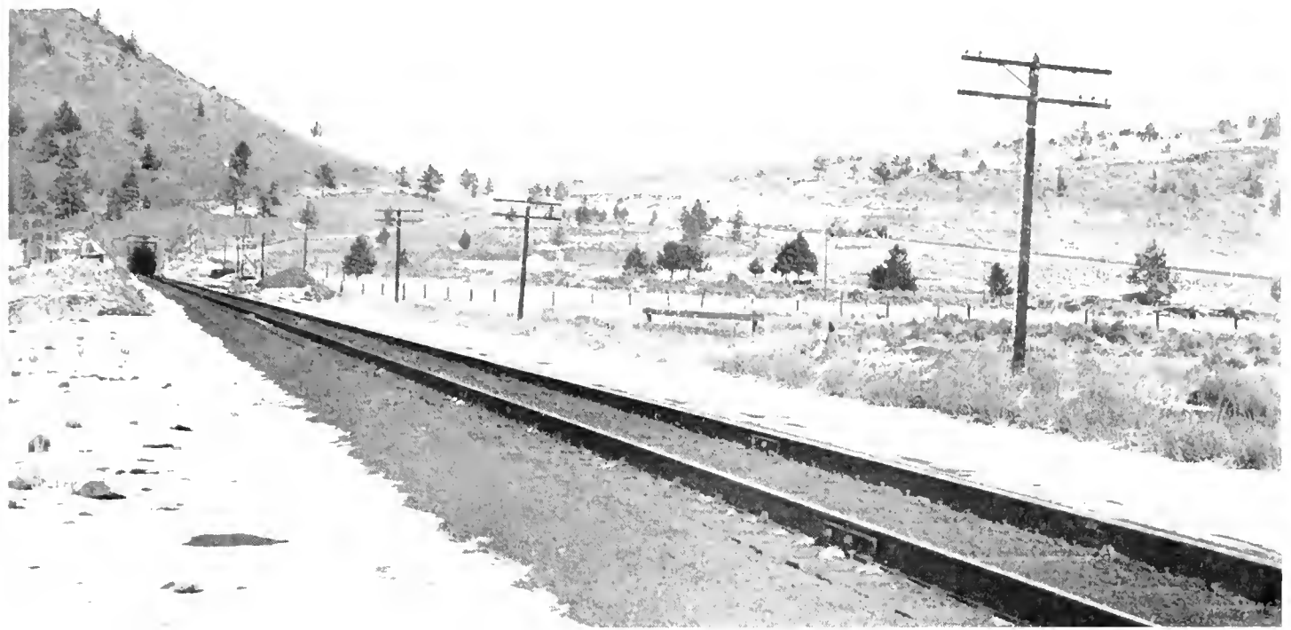
Showing railway tunnel at the left, with highway passing through cut in center background
